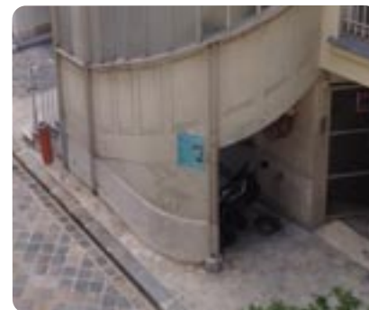
• Staircase on courtyard, with access to cellar
